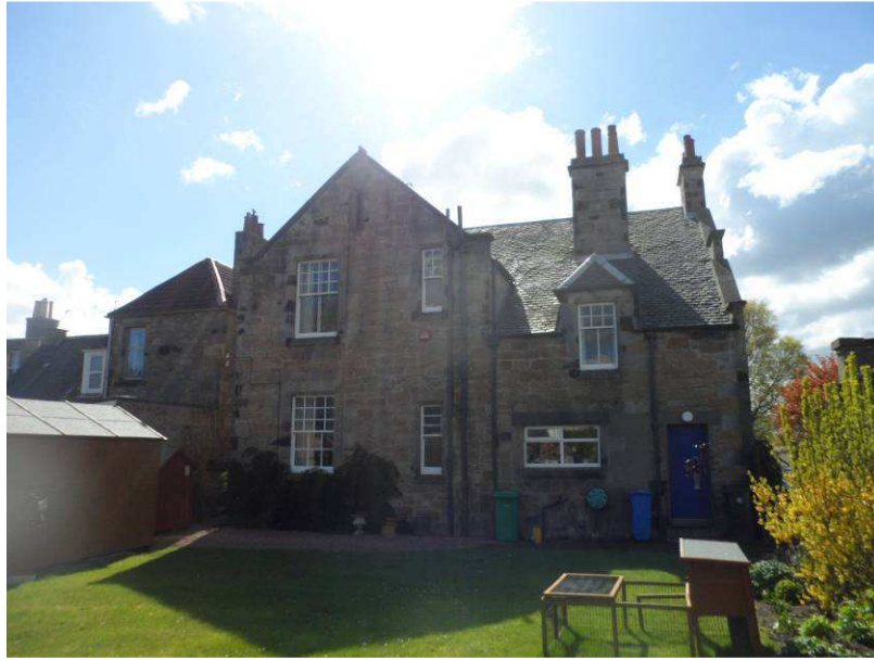
General view of rear elevation
