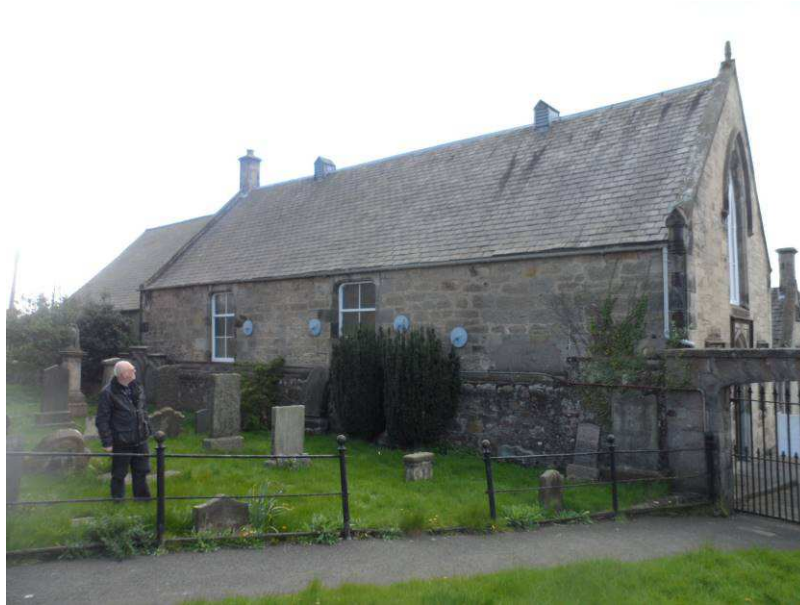
General view of rear elevation
