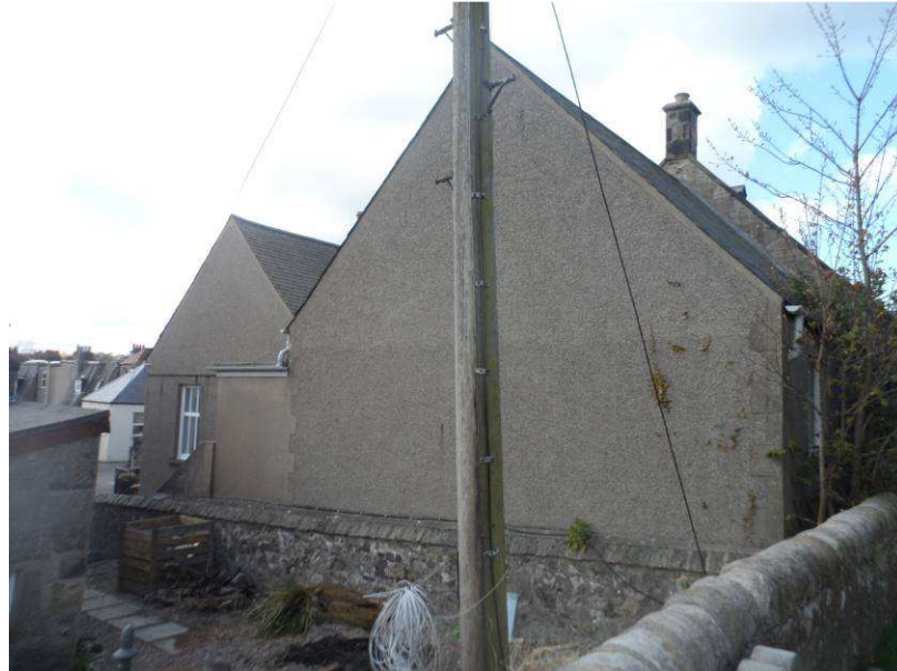
General view of east elevation
