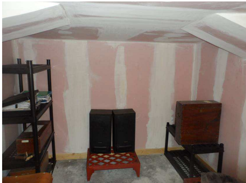
View of new safe within basement
