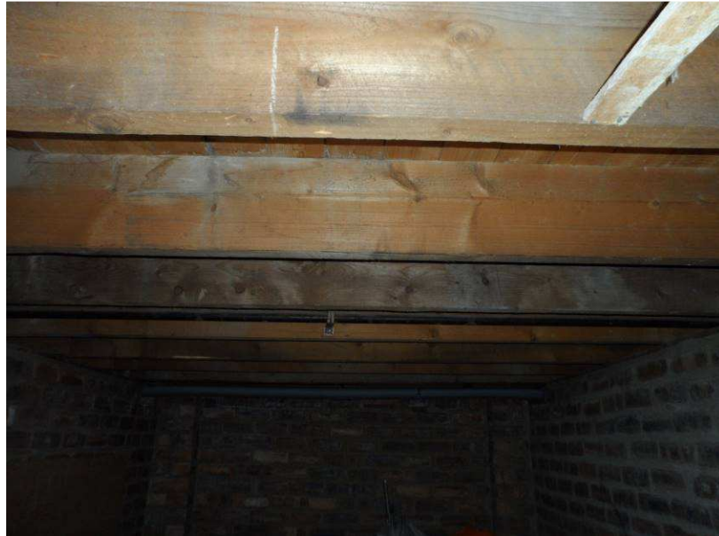
View of timbers within basement
