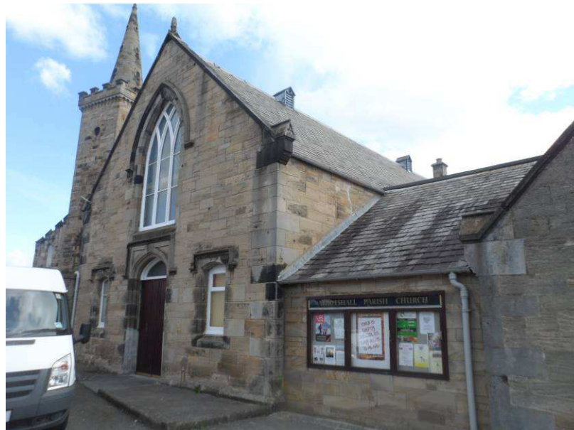
General view of west elevation
